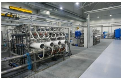
TESTING OF ELEMENTS
